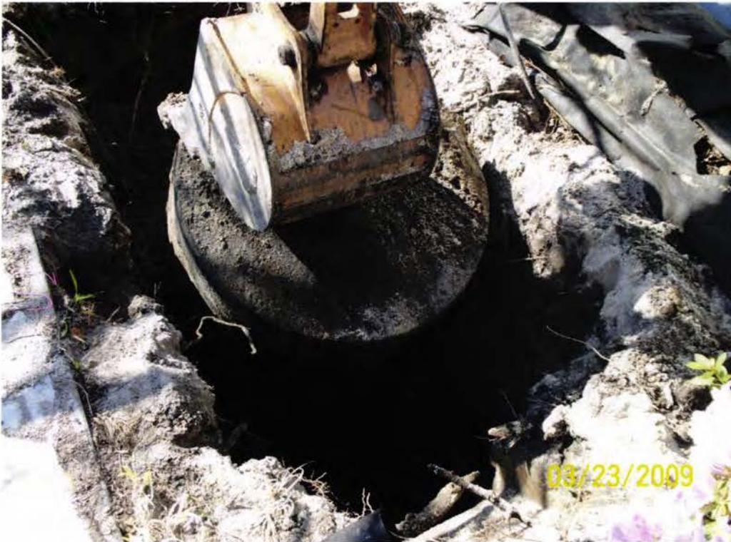
Picture 2: UST 152 Laurel Bay Blvd being removed from the excavation.
